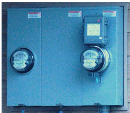
Underground or overhead style 2 position meter base
