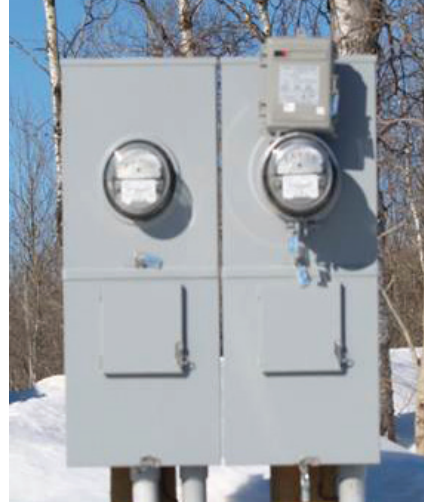
Minnesota Power underground lot line meter base installation
