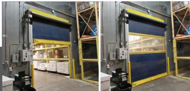
High speed automatic doors on coolers and freezers keep cold air from escaping, resulting in significant energy savings.
