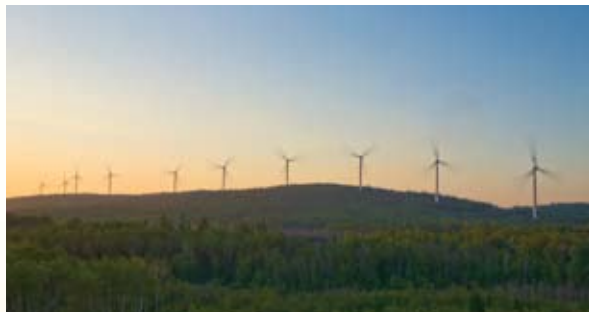
Minnesota Power's Taconite Ridge in Northeastern Minnesota creates enough energy to power 8,000 homes a year.
