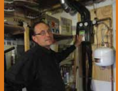
An evacuated tube solar thermal water heating system meets more than half of the Johnson’s annual hot water needs.
