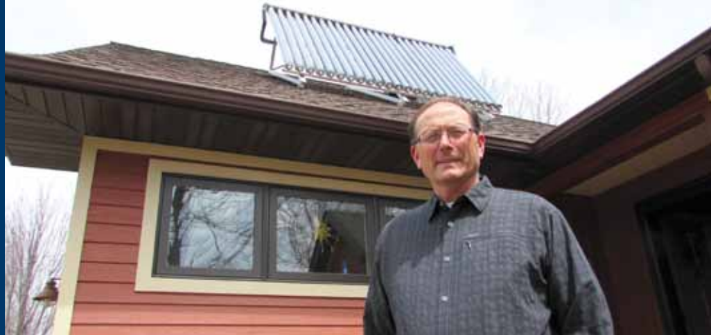
David Johnson uses a solar thermal water heating system with an electric backup in his home.
